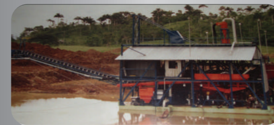
Washing Plant for Alluvial Gold - ECUMINAS
