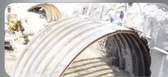
Trusses Guayasamin Tunnel - CARTELLONE
