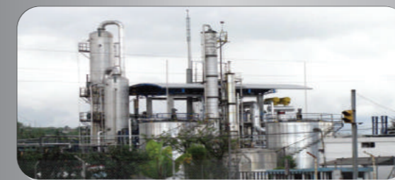
Industrial Plant - INTERQUIMEC
