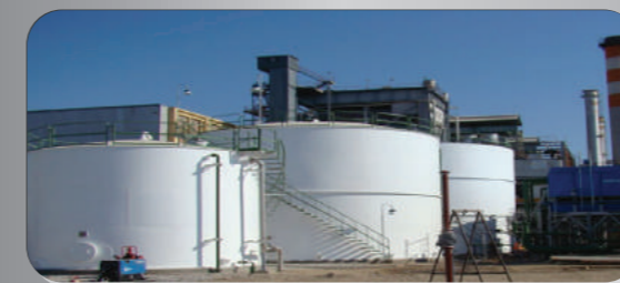
Guemes Thermal Power Station - PAMPA ENERGIA
